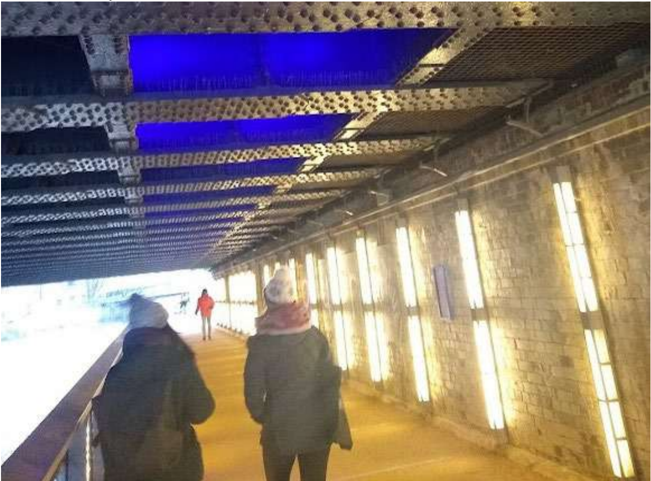
Figure 16. Lighting / art installation on canal underpass.
